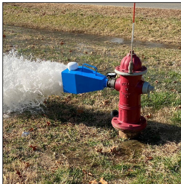
Fire Hydrant Flushing at Naval Support Facility Dahlgren. Source: NSFDL Stock Photo
